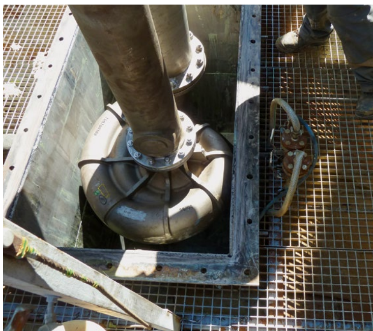
The vertical pump is installed in the tank of the sulphuric acid plant.
