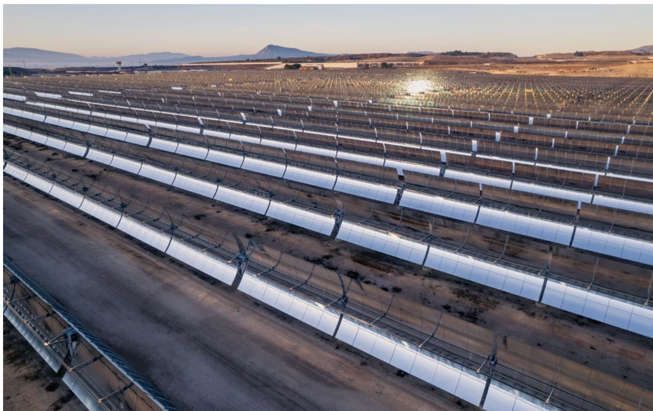
Parabolic reflectors bundle the sunlight and effectively focus the solar radiation onto a receiver pipe.
