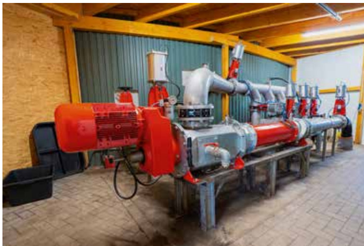
To convey the liquid phase to the liquid feeding system, the operators of the biogas plant installed the progressive cavity pump with its conical rotor-stator geometry.
