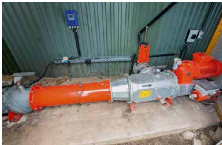
For the external heat exchanger, the biogas plant operators used the automatic version of the conical progressive cavity pump.
