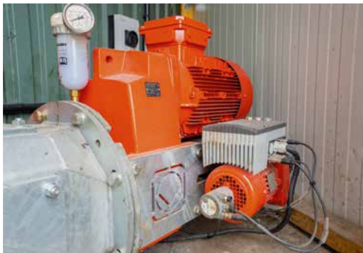
The progressive cavity pump running on the heat exchanger is particularly energy-efficient thanks to the automatic start-up feature.
