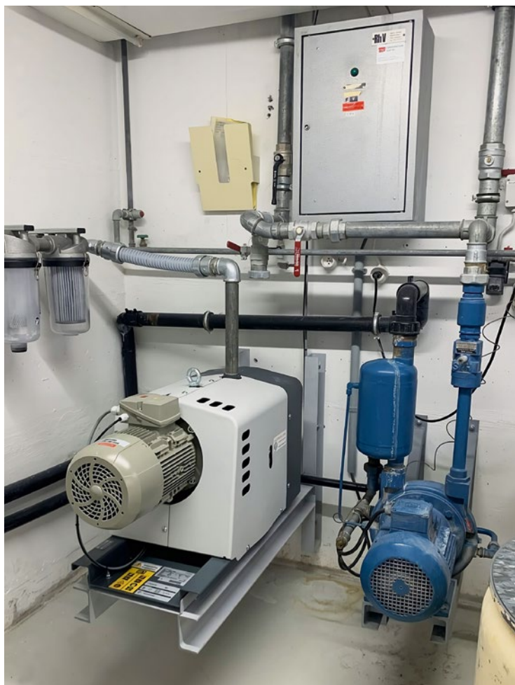
A claw pump replaces the liquid ring pump when mixing and degassing multi-compounds resin.
